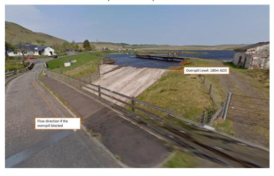
Photo 7: Overspill of the compensation reservoir
